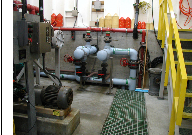
Figure D7: Filtered Cold Seawater Transmission Piping
